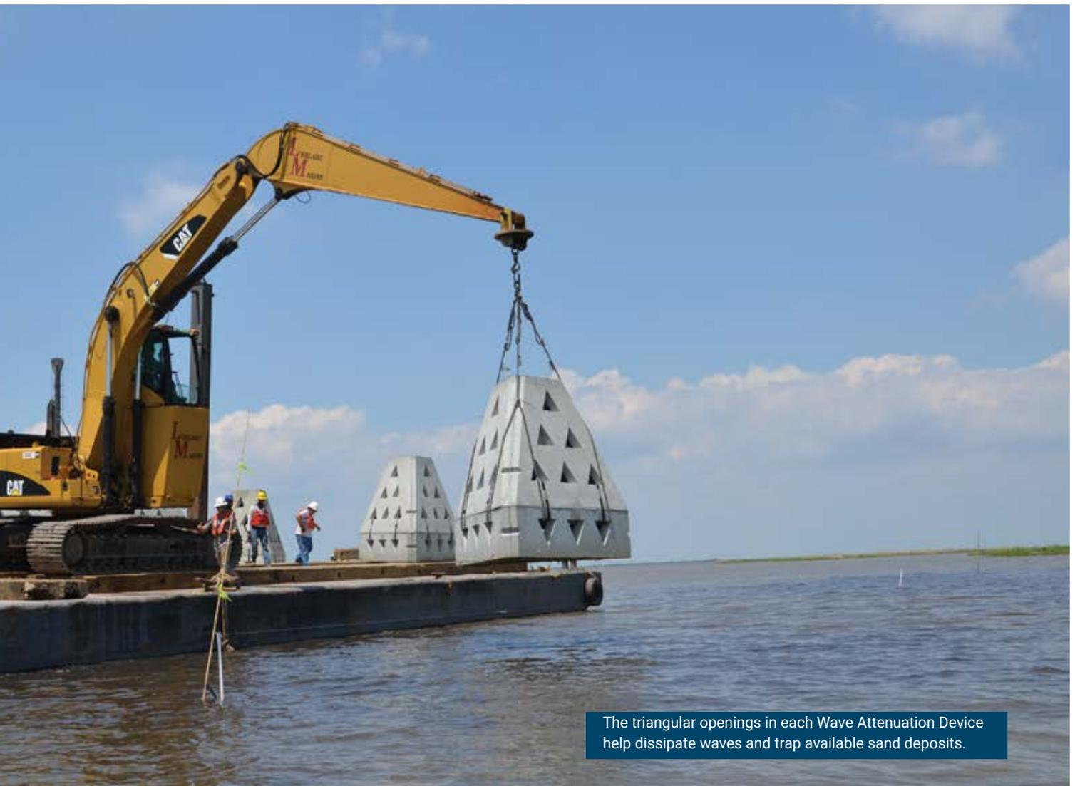
The triangular openings in each Wave Attenuation Device help dissipate waves and trap available sand deposits.
