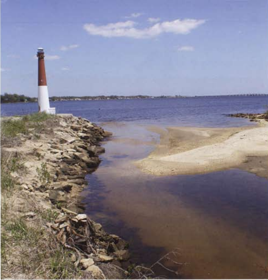
This lagoon had been filling up with sand. Beach prisms have helped to keep the sand from flowing out of the river.
