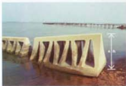
Beach Prisms work by reducing the amount of energy in incoming waves before the waves reach the shoreline. Waves pass through the specially designed slots.
